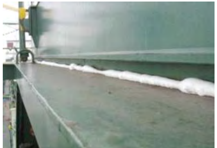
^ The use of foam is not a primary means of preventing water ingress v
