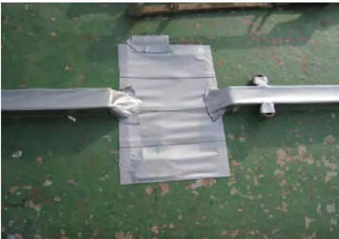
^ v The use of tape is not a primary means of preventing water ingress
