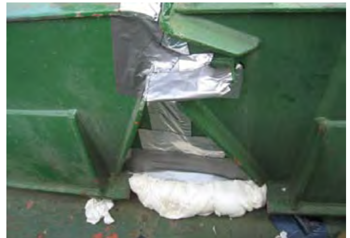
^ The use of foam and tape is not a primary means of preventing water ingress
