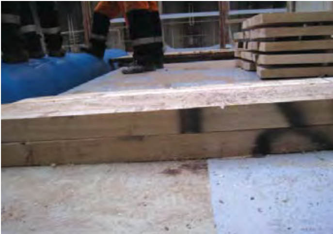
^ Use of ample dunnage protects the cargo
