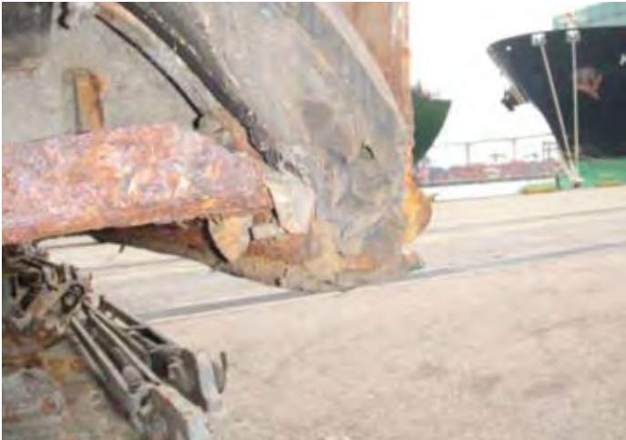
^ Damaged container ship hatch corner rubbers would allow water ingress
