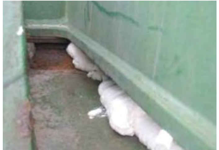
^ The use of foam is not a primary means of preventing water ingress v
