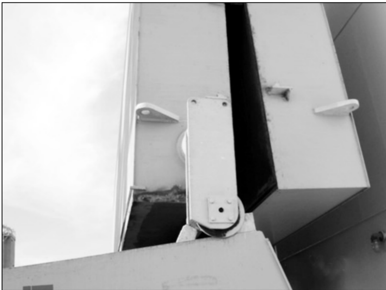
Attention to detail: particular care is taken to ensure the hatches are in proper working condition.
