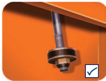
Cleat – washer in good condition
