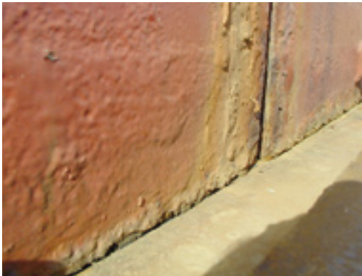
Panels resting freely onto coaming.
