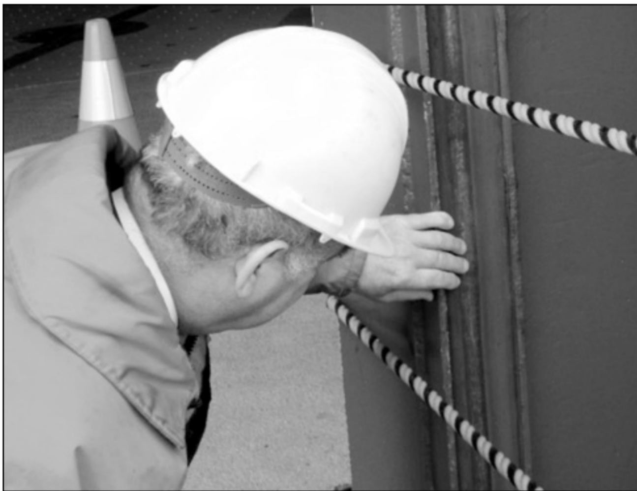
Seal of approval: the ship inspector checks rubber seals on a car carrier stern ramp.
